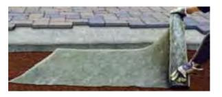
Air and water can pass through landscape fabric preventing soil loss, reducing weeds and maintaining more even soil temperature.
