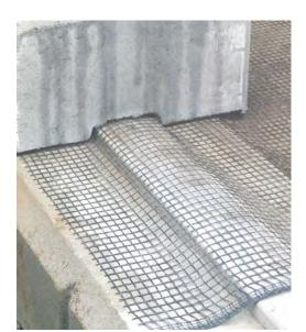
A geogrid is a mesh-like system integrated into the construction of driveways and retaining walls to reinforce soil & gravel by providing additional support and redistributing the weight of pressure placed on the surface, across a wider area. Geogrids are manufactured using polymers (polyester, polyethylene) known for their tensile strength and durability.
